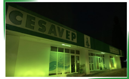
Facilities of the Puebla Plant Health State Committee
